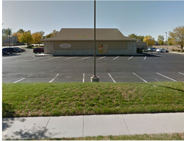
One-story church south of the subject site, facing south from E. Elk Drive.
