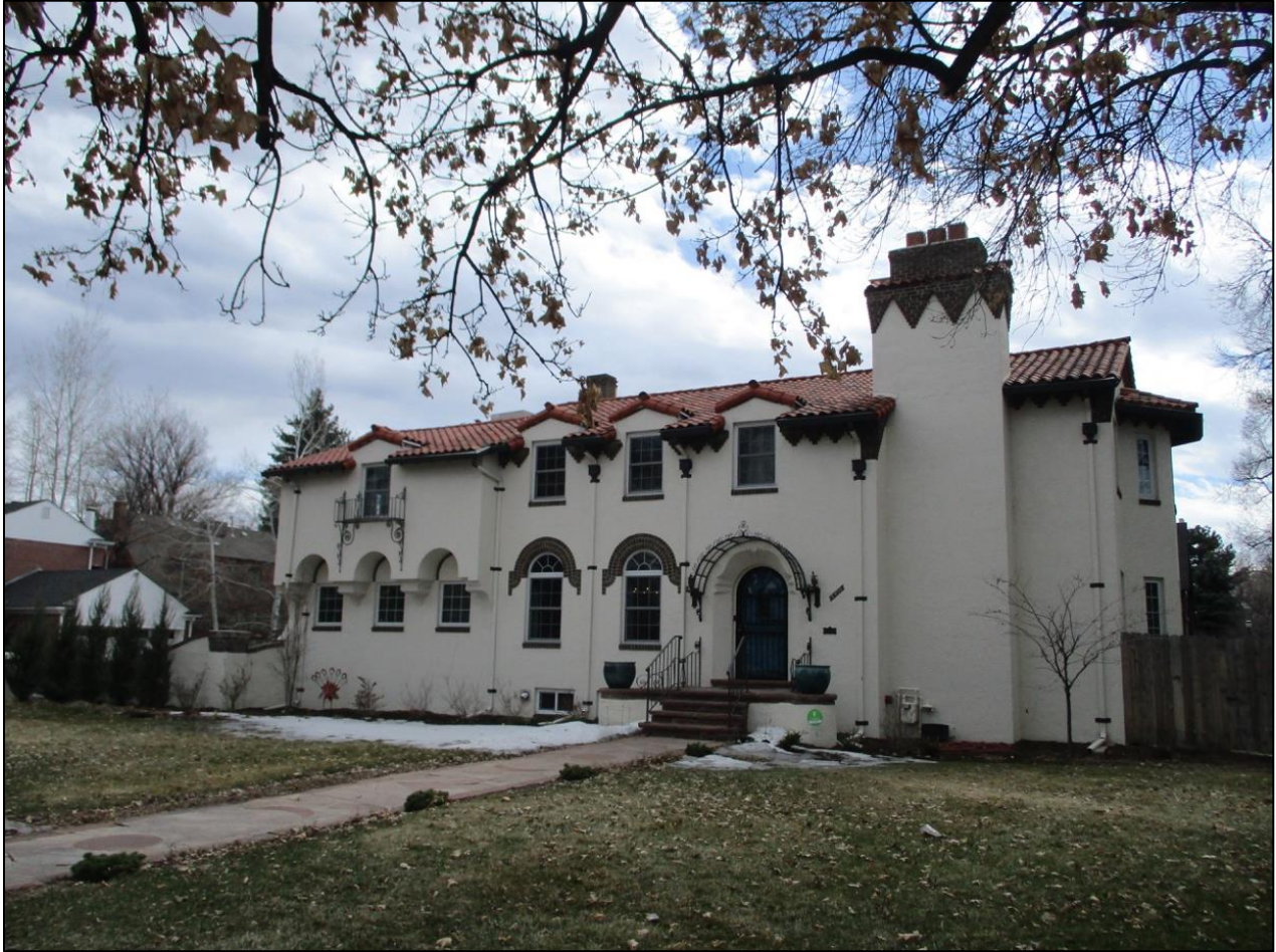
Figure 1 Looking southeast at the primary facade of 6400 Montview Boulevard
