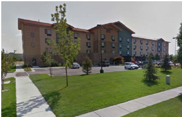
Mid-rise lodging to the west of the site
