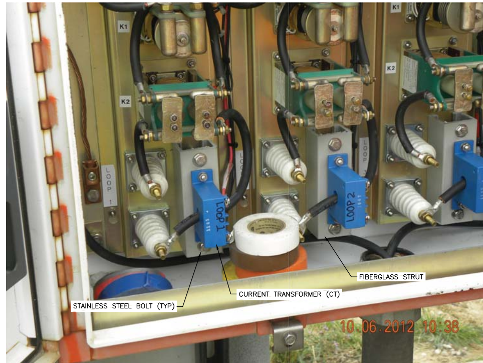
1 PROPOSED CURRENT TRANSFORMER (CT) INSTALLATION NTS
