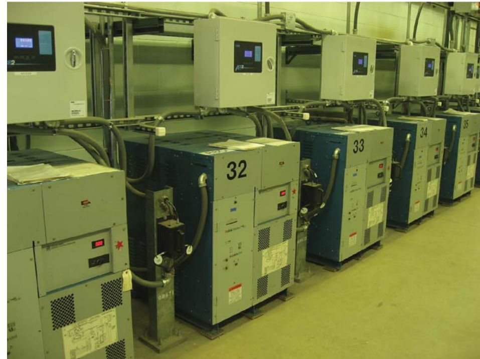
2 EXISTING CCR INSTALLATION NTS
