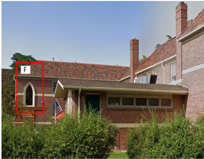
Figure 1-4: Facade Feature F
