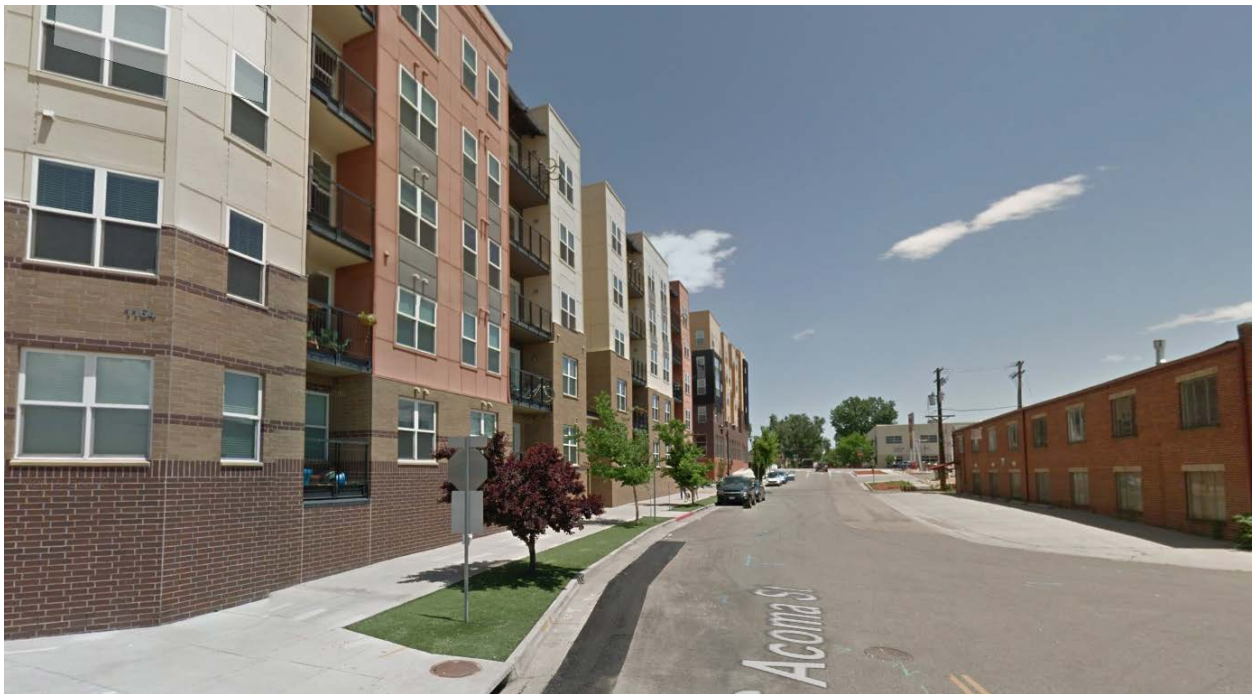
Subject site at the intersection of S. Acoma St. and W. Arizona Ave looking east
