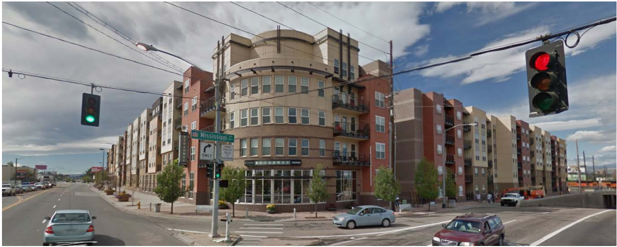
Subject site at the intersection of S. Broadway and W. Mississippi Ave. looking southwest
