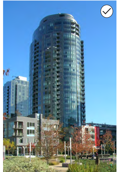
An example of a point tower in Portland, Oregon.
