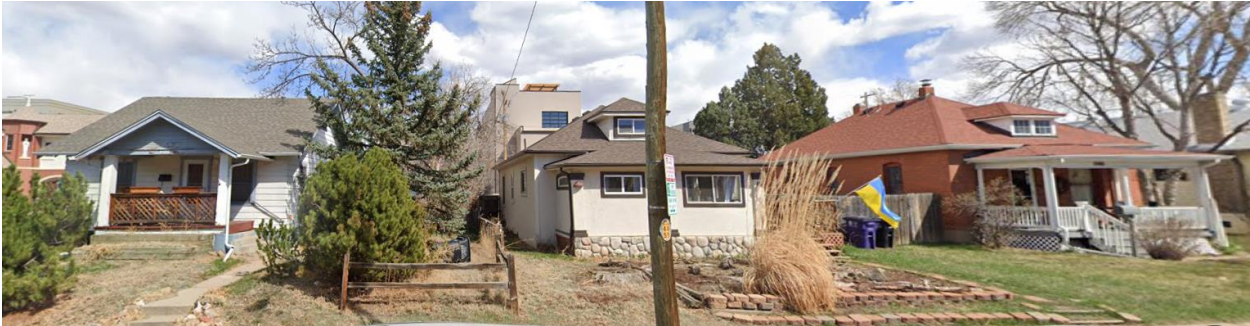
View of the properties to the south of Holy Family Church and east of Arrupe, looking east from Utica Street
