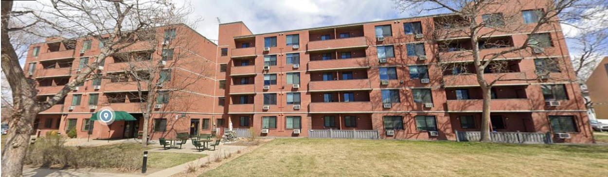
View of the property to the west of Arrupe, looking east from Vrain Street.
