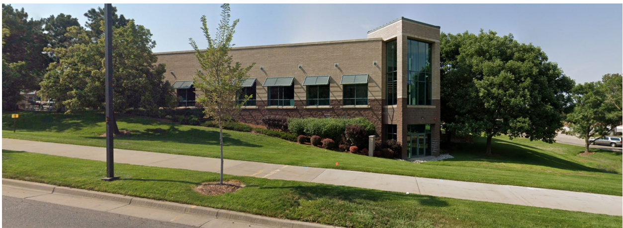
Site (8351 E. Belleview Ave.) – from East Belleview Avenue (Source: Google Maps)
