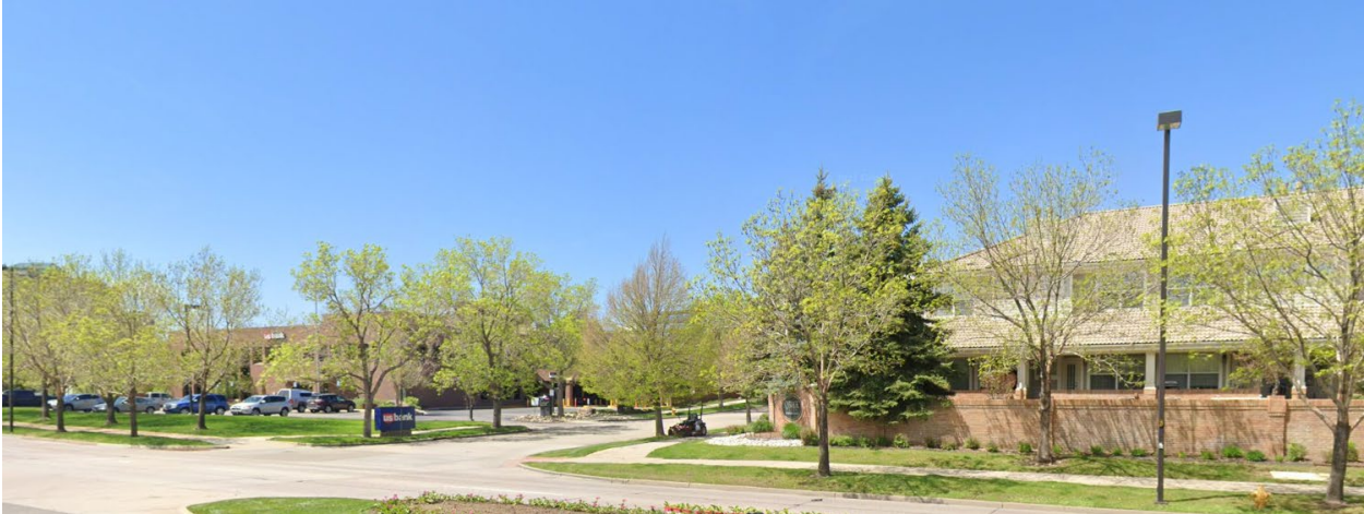
East – from DTC Boulevard (Source: Google Maps)
