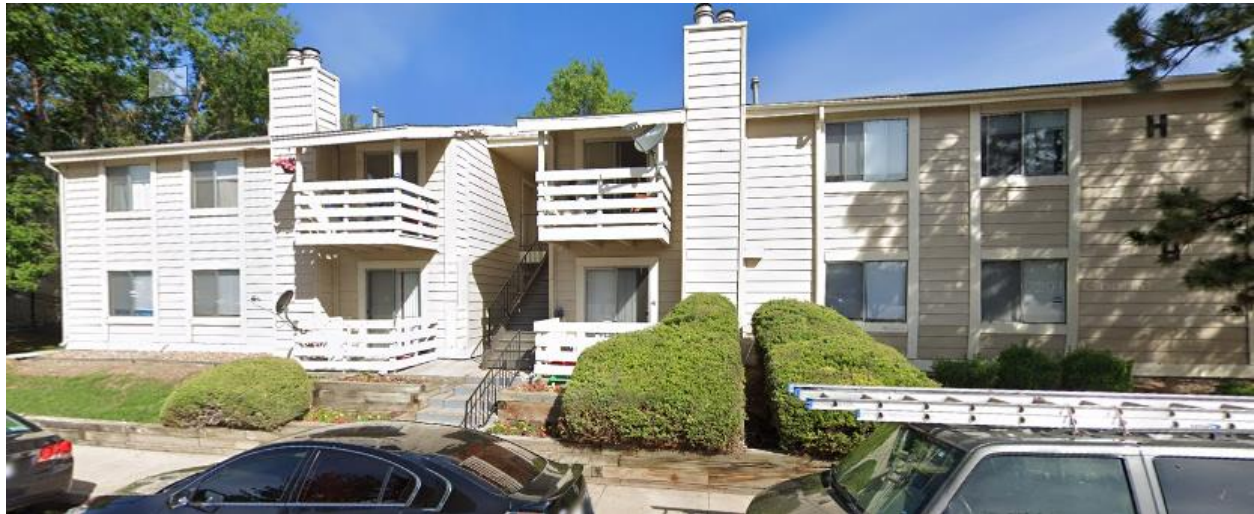
View of the property to the south, looking north.
