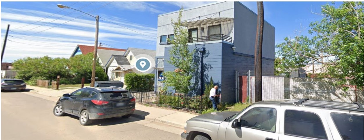
South – from South Acoma Street (Source: Google Maps)
