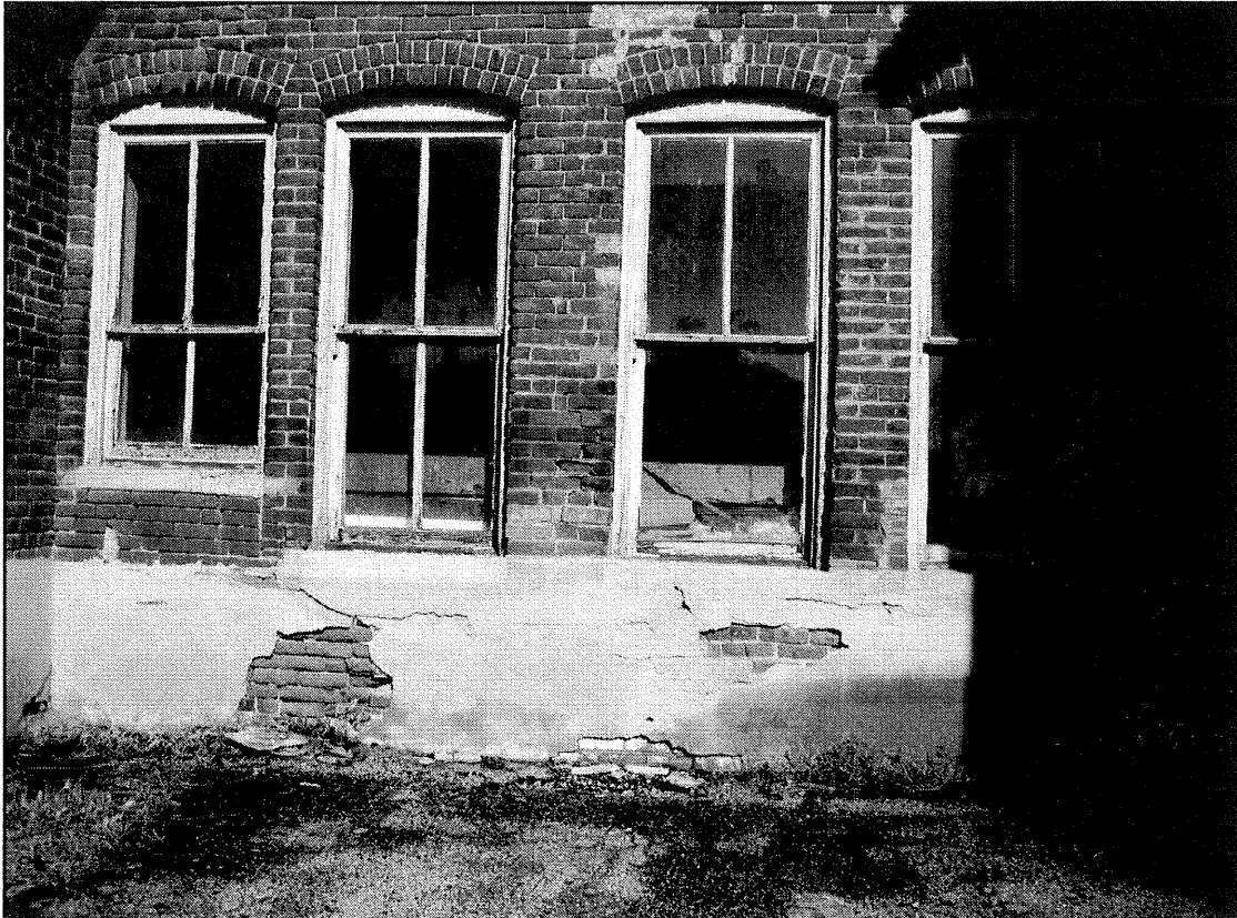
Figure 2-1: Deteriorated Wall
