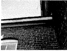
4_Deteriorated Fascia_Soffits.jpg
