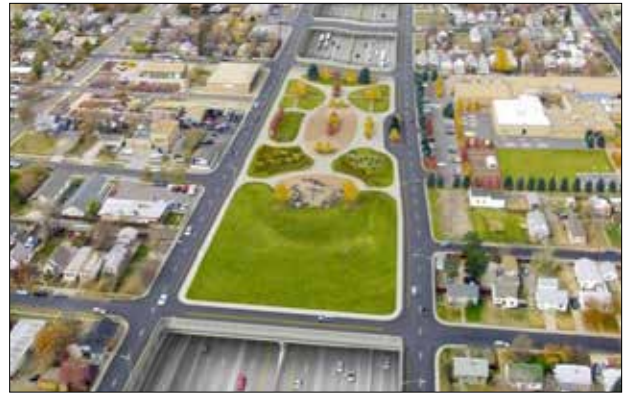
The I-70 East project will be reconstructed between Brighton Boulevard and Colorado Boulevard with a lowered segment of the highway. A new covered park is proposed at Swansea School.
