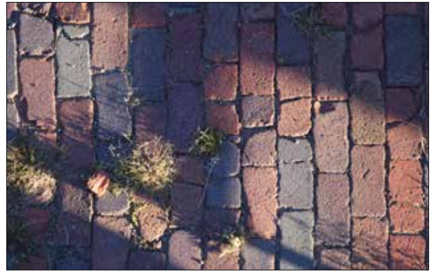
The brick pavers in the existing yards are an important historic artifact that will be reused in the new NWC.
