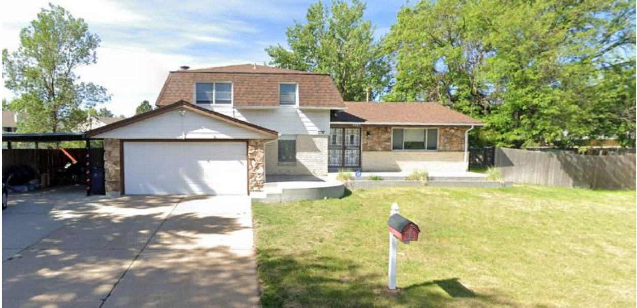
View of property looking south.
