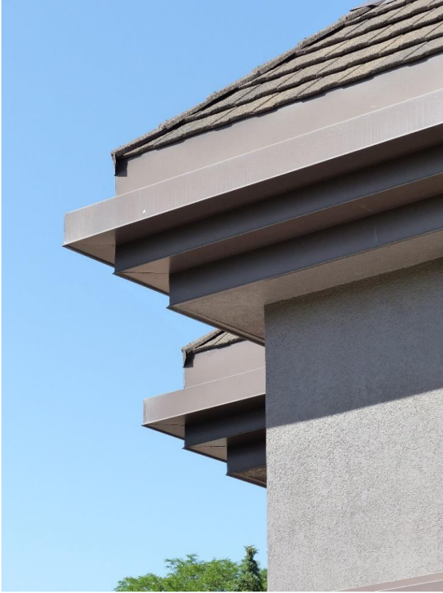
Figure 21: Detail of eaves showing corbelling
