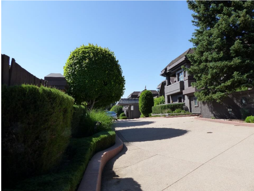
Figure 13: Driveway running along the façade of Cableland, looking northwest
