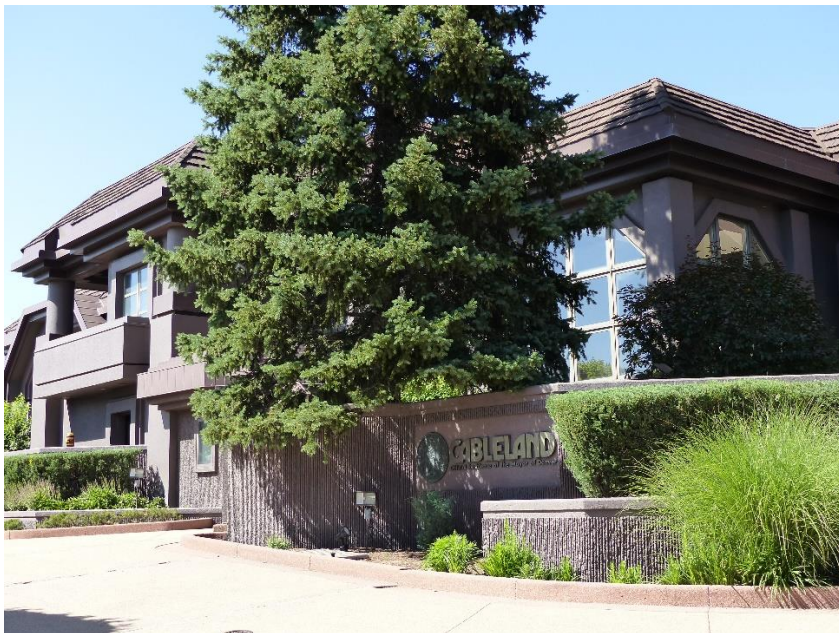
Figure 14: Façade, looking north
