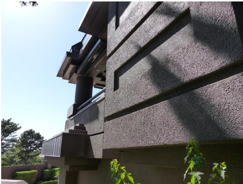
Figure 20: Southeast side of house showing recesses in wall and recessed balcony
