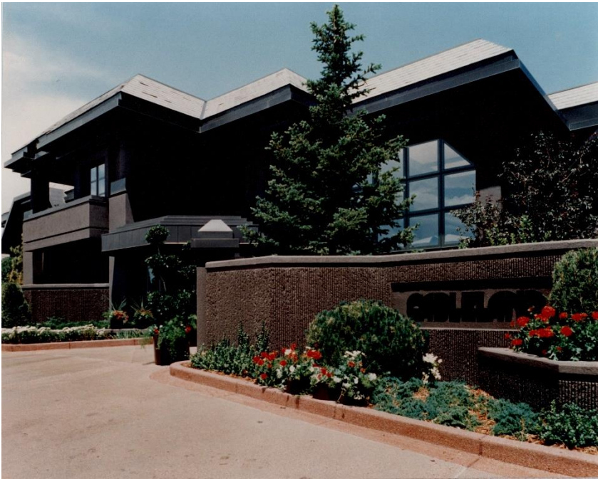
Figure 1: Façade, looking north
