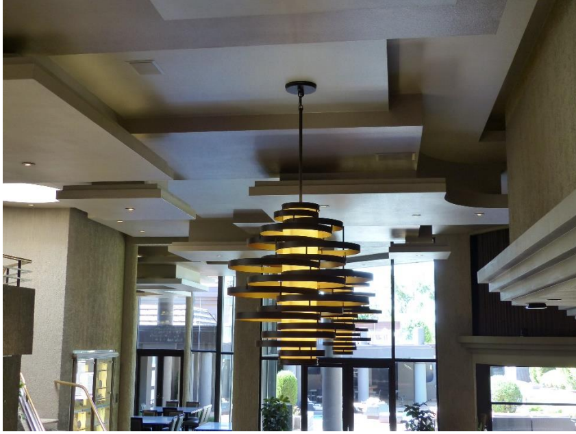
Figure 29: Reception area, detail of dropped ceiling panels
