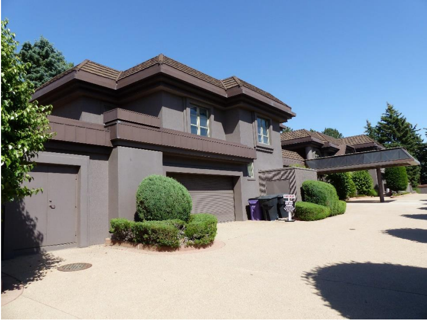
Figure 17: Façade of cabana and guest house, looking east
