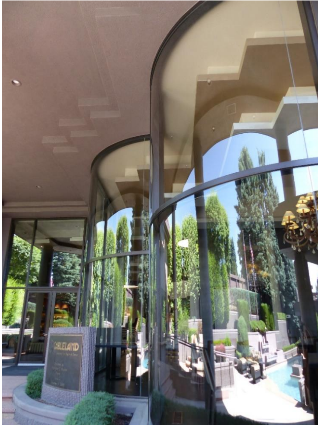
Figure 27: Courtyard, detail of curved glass walls and corbelling at main residence
