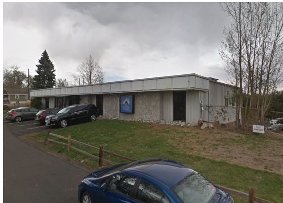
East – Delaware St.
