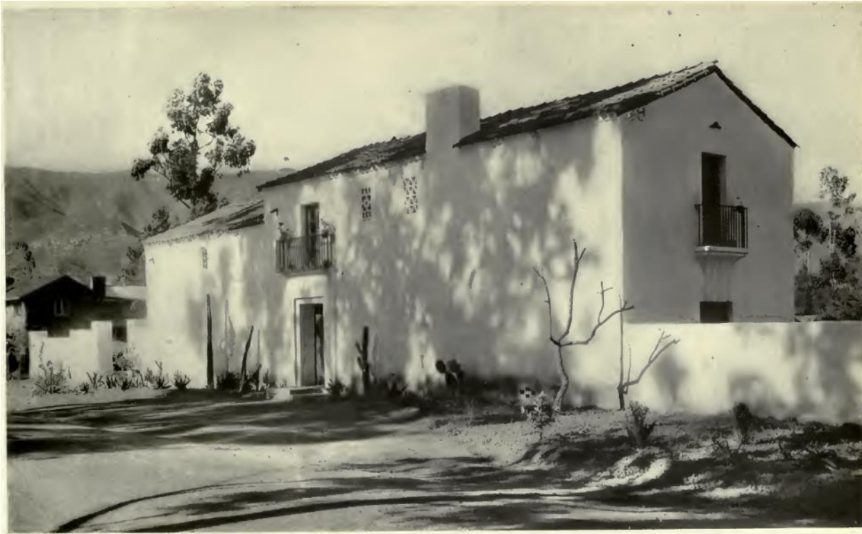
ENTRANCE SIDE--"CASA DRACAENA," RESIDENCE AT SANTA BARBARA, CAL., OF GEORGE WASHINGTON SMITH, ARCHITECT.
