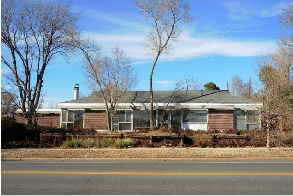
2600 Milwaukee, south elevation. Image by Shannon Stage, 2018.
