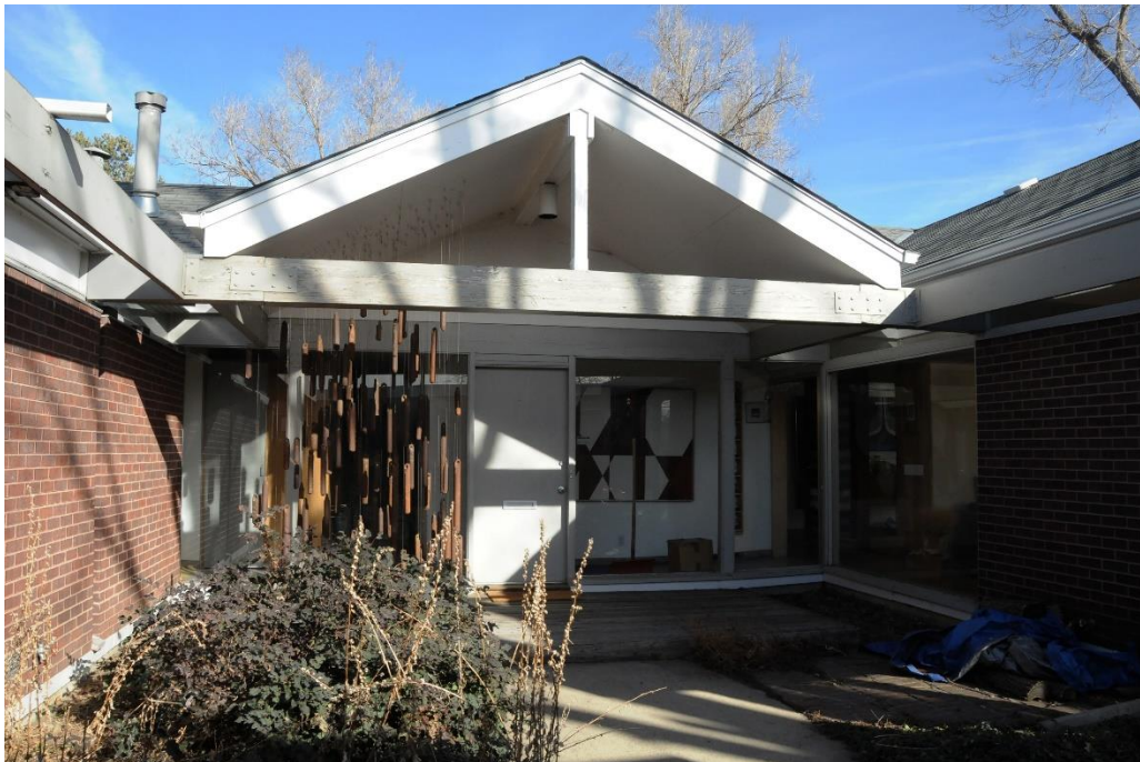
2600 Milwaukee, recessed entrance. Image by Shannon Stage, 2018.
