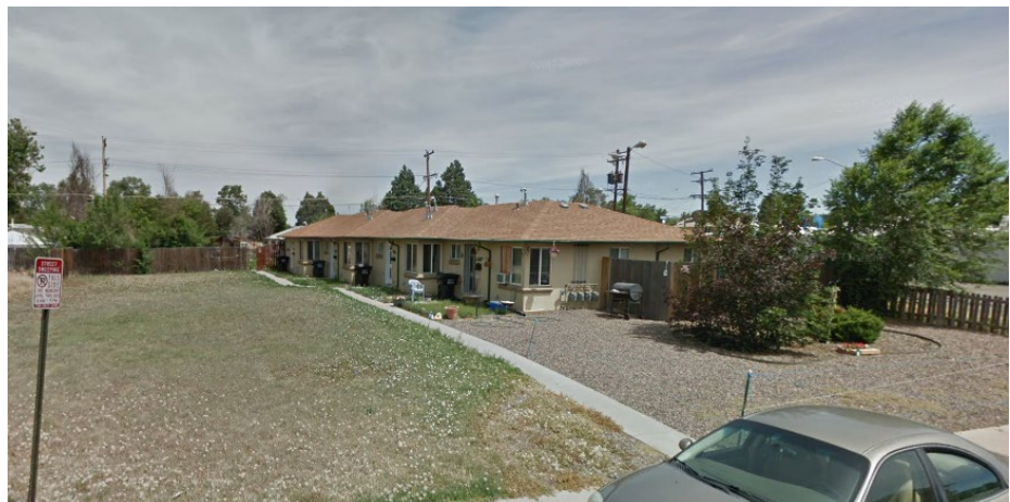
View of property to the north of the subject site on Valentia Street, looking east
