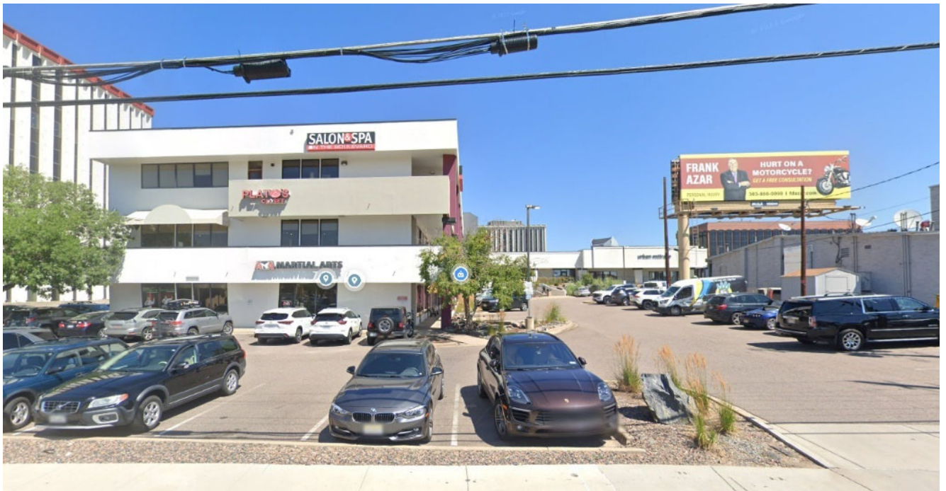
East - The property to the east, looking north from East Florida Avenue
