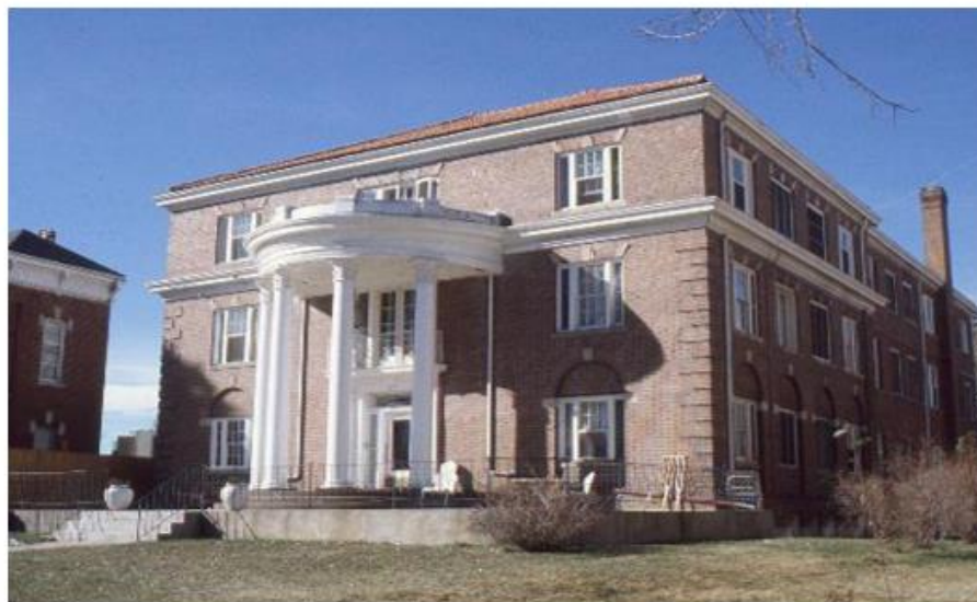
Photos: Patients Building ca. 1924-25 and 2018.
