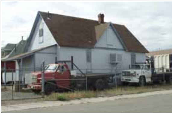
Housing converted to industrial storage yard
