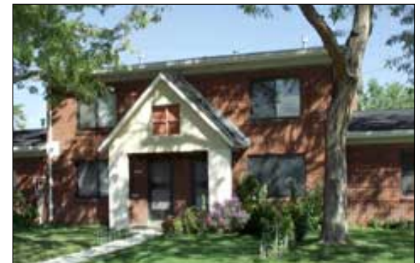
Recently renovated Quigg Newton homes
