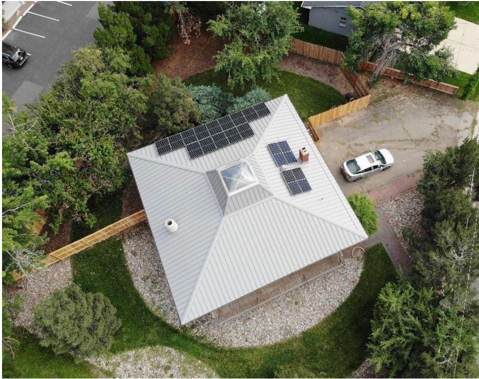
An aerial view of the standing seam roof and photovoltaic solar collectors on 602 S Harrison lane.
