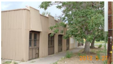
Figure G – Existing facade
