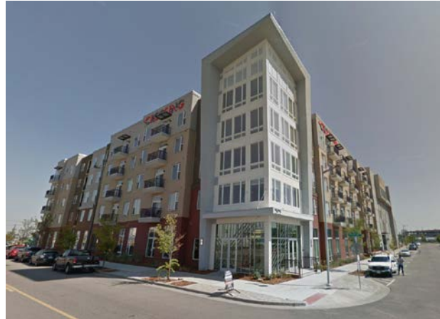
North – at Denargo St. and Wewatta Way
