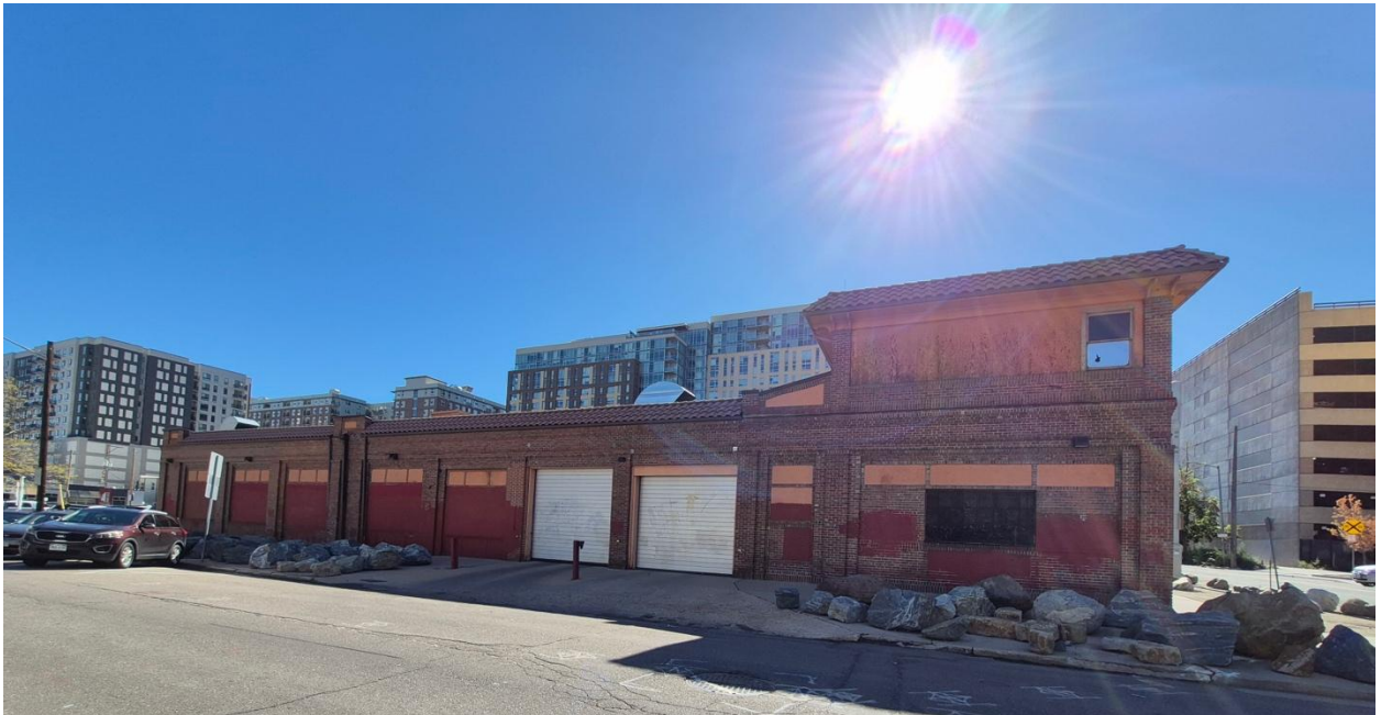
California Street Garage, northwest elevation (2025)
