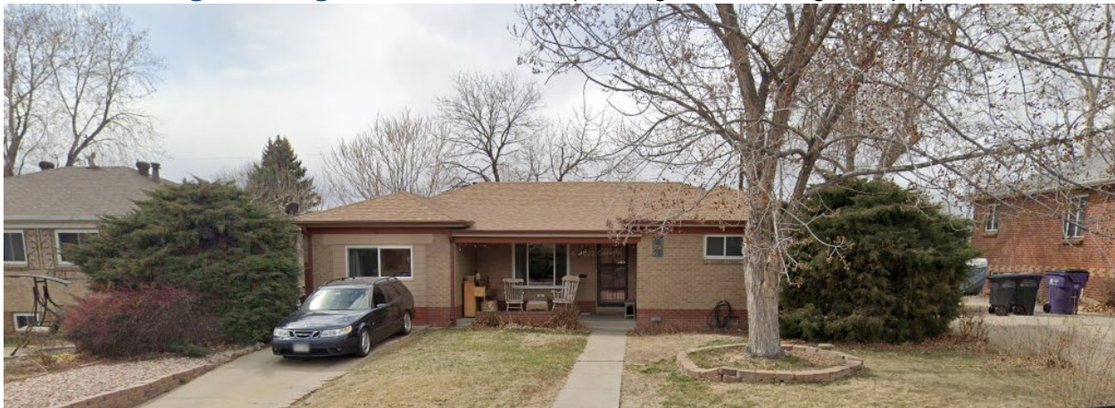
Subject Site - View of the subject property, looking east.
