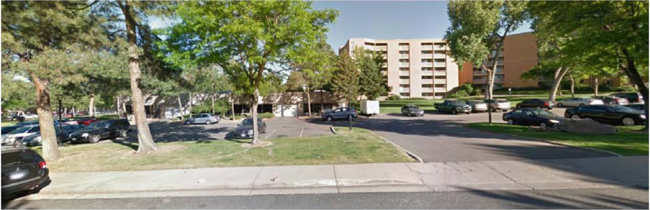
Woodstream Village Looking West
