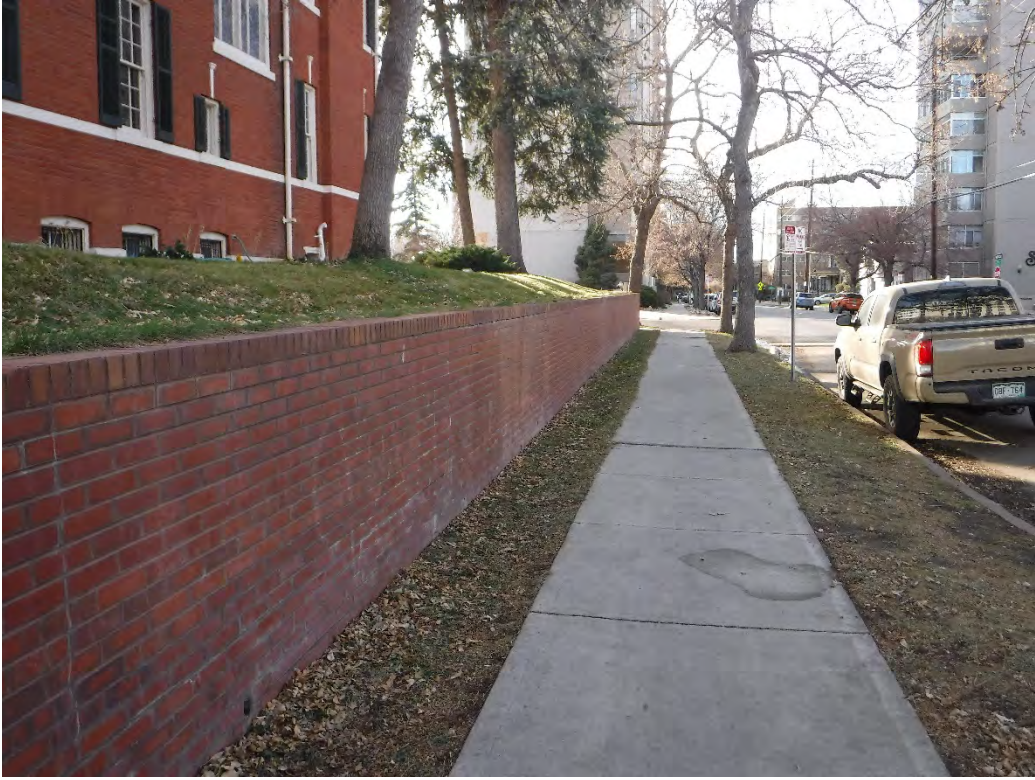
15. Brick retaining wall on north side of the Tears-McFarlan House.
