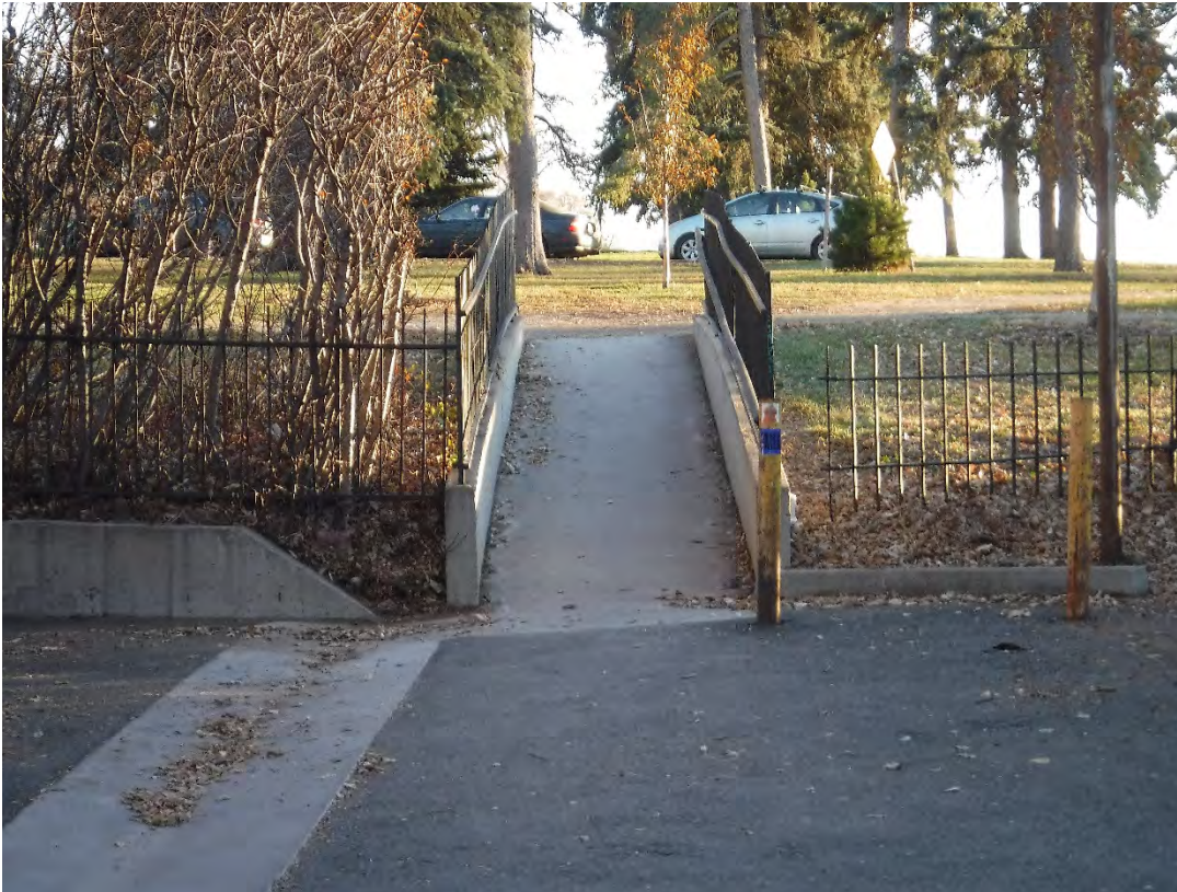
6. Williams Street access ramp to Cheesman Park (looking south).
