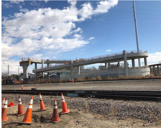
47th & YORK PED BRIDGE
