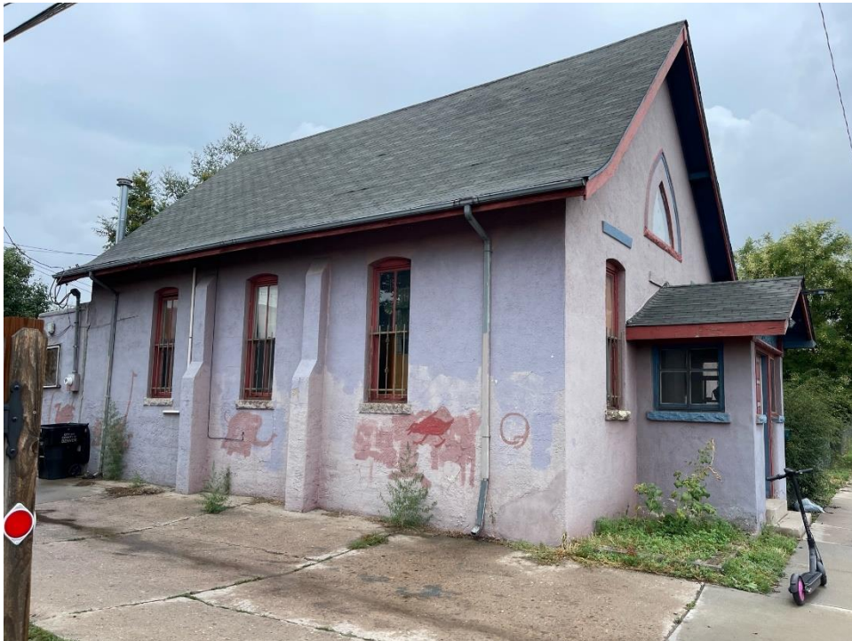
North and East Facades of 1618 E. 38 th Ave.
