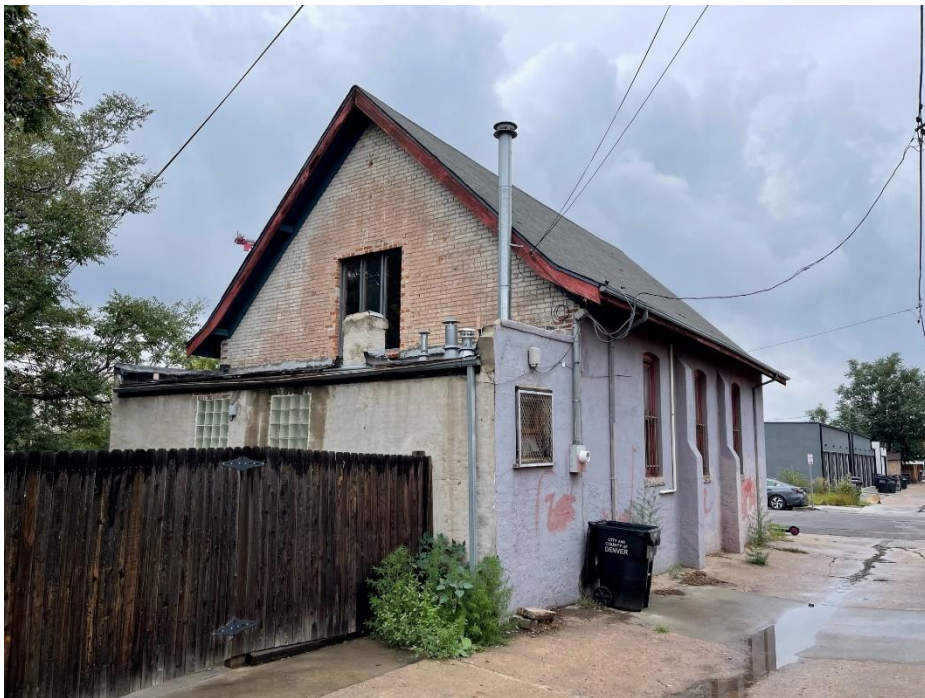
South Facade of 1618 E. 38 th Ave.
