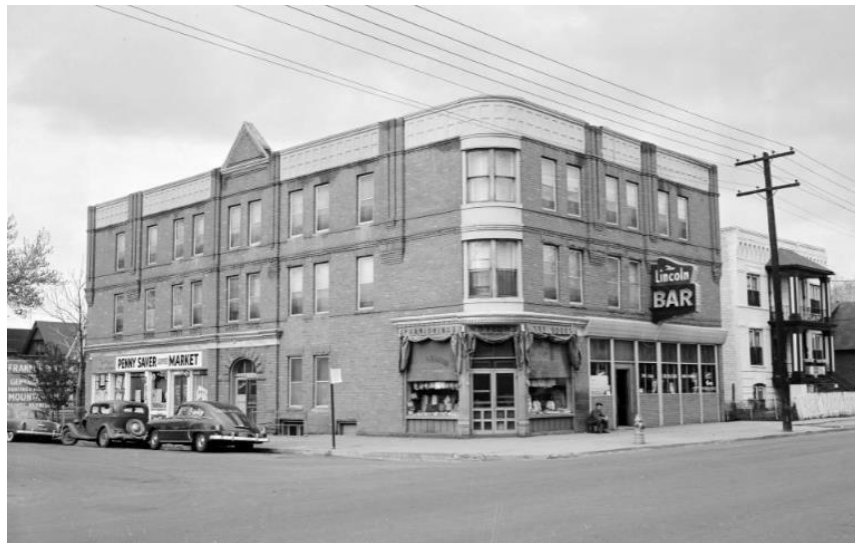
Figure 7 – This substantial two-part commercial block building at Franklin Street and Bruce Randolph Avenue was built in 1890 and designed by architects Kidder & Humphries. The ground floor had a drug store, barber shop, and a bar, while upstairs were apartments. Denver Public Library Digital Collections photograph.
