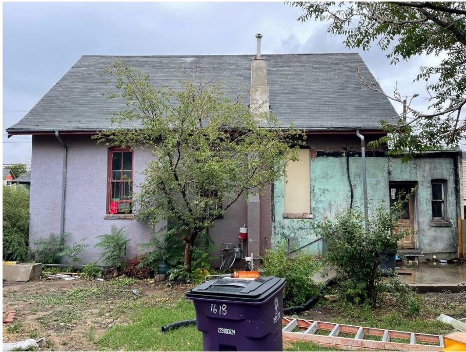
West Facade of 1618 E. 38 th Ave.
