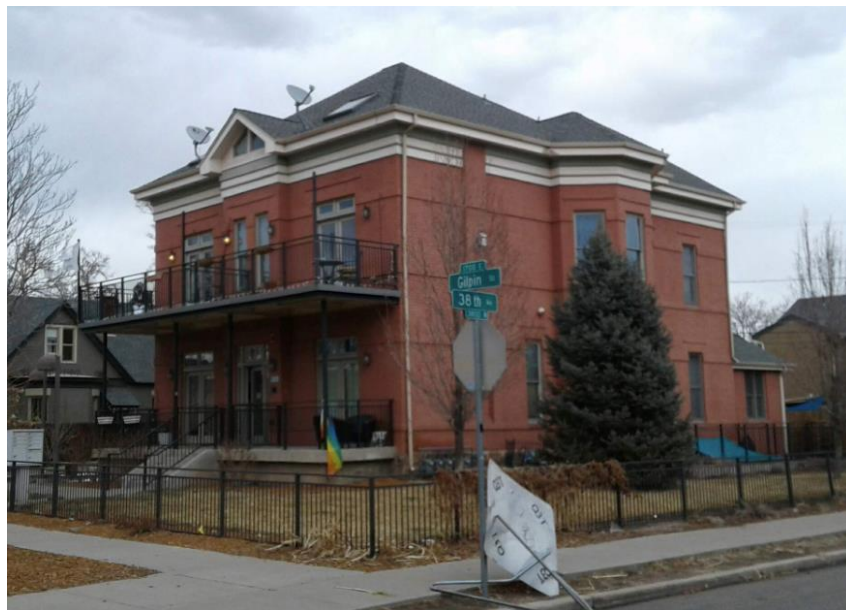
Figure 4 - The David Rubidge house at 3800 Gilpin Street was built in 1890. Discover Denver
