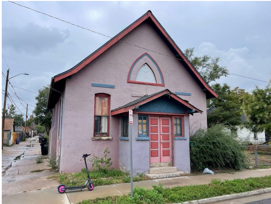
North Facade of 1618 E. 38 th Ave.
