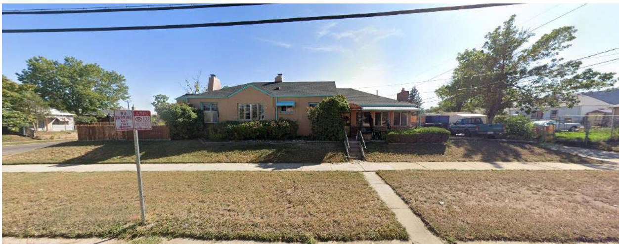
Site – Subject property, looking south from 5 th Avenue
