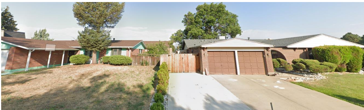
View of single-family residences to the east of the subject site, looking west from North Quentin Street.
