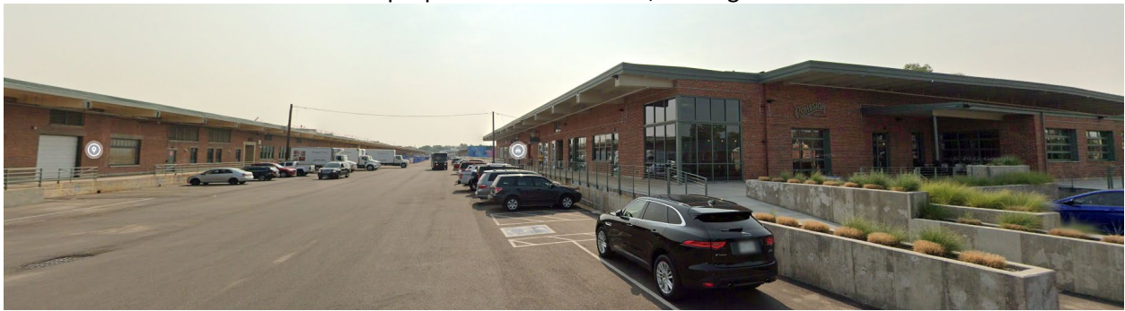
West - View of the York Street Yards properties from the west, looking southeast.
