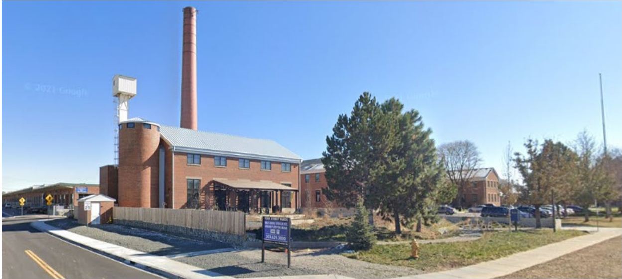
View of the northern portion of existing PUD-G 32 from the west.
