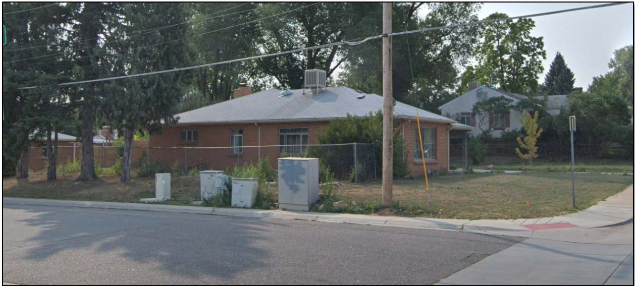
Figure 6f: View of Property Across E. Iowa Ave. to South
