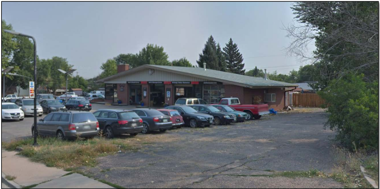
Figure 6c: View of Adjacent Property to North
