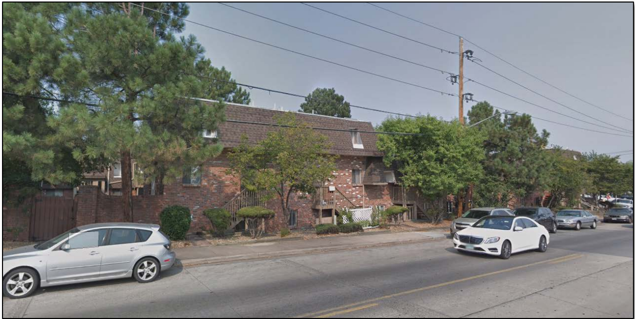
Figure 6d: View of Multi-Unit Development Across S. Holly St. to West
