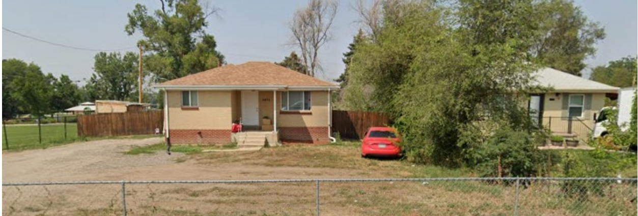
View of the property directly east of the subject site, looking north from W. Kentucky Ave.
