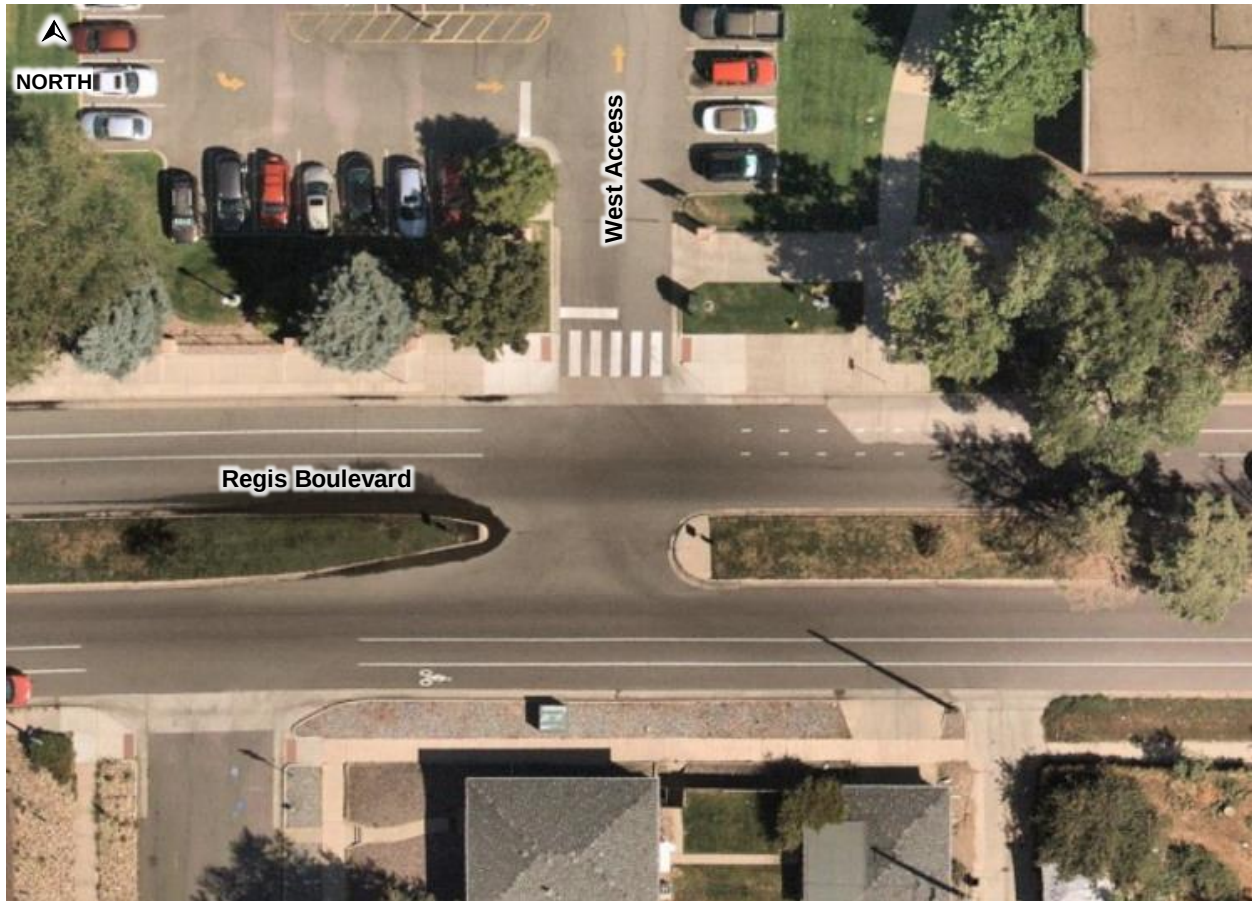
Regis Boulevard West Access (#6)
