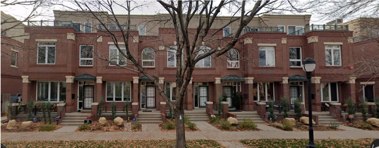
View facing east on Garfield Avenue south of Ellsworth Avenue
