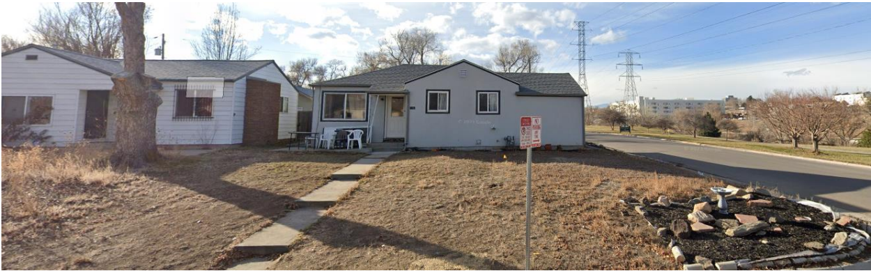
West – Properties to the west of the subject site on North Hooker Street.
