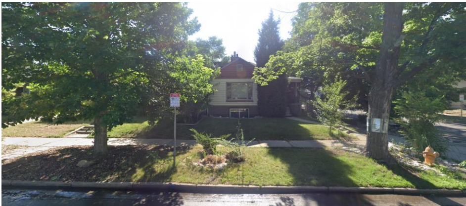
1896 S Humboldt St. - View of the subject property, looking east from South Humboldt St.
