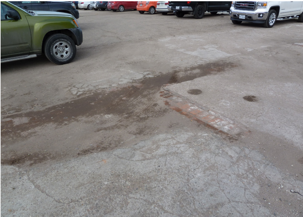
Potholes and remnants of building foundations and railroad tracks still exist in places on the uneven parking surface
