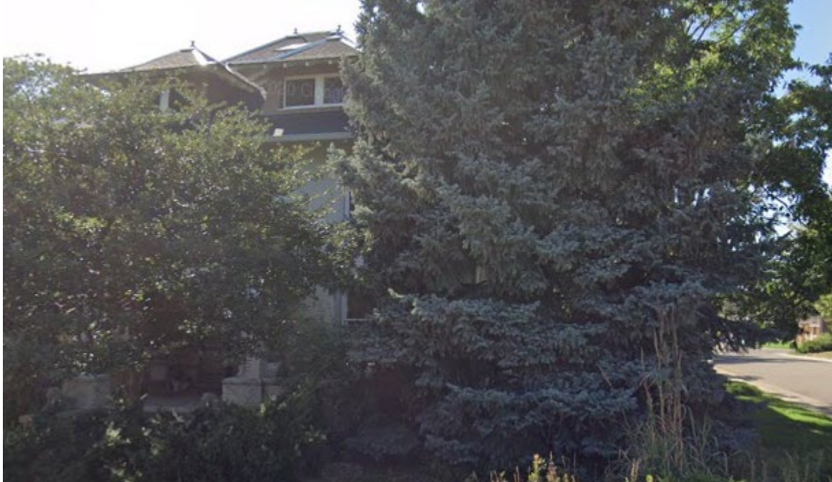
View of the property to the south looking west.
