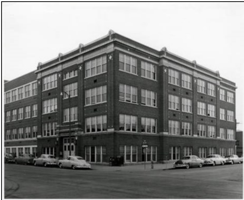
12. Photo of original 1926 schoolhouse. Photo c. late 1940s. Courtesy of Denver Public Library. This photo shows the building’s original entry doors and wood sash windows.
