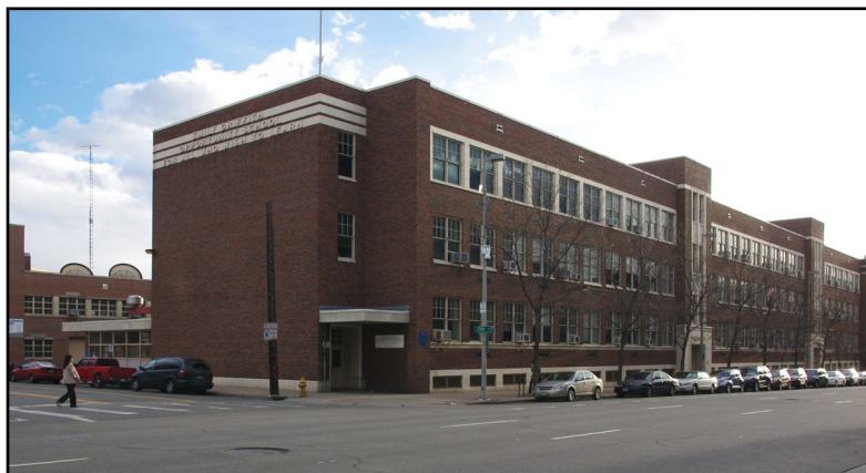
5. View of the school from Welton and 13th Streets. The historic structure conveys its massing, volume and form as a distinct entity.
