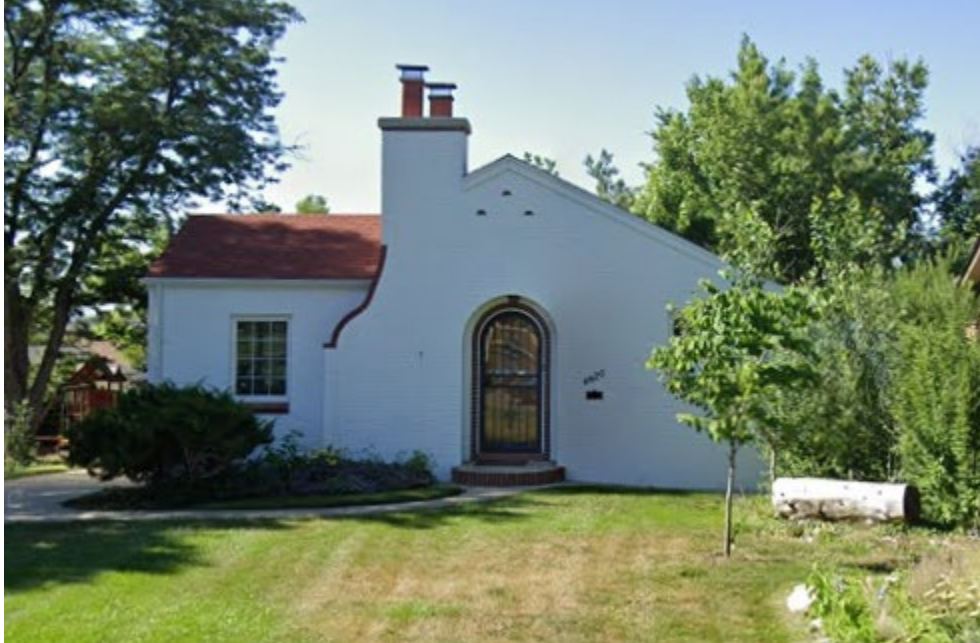
View of property looking south.
