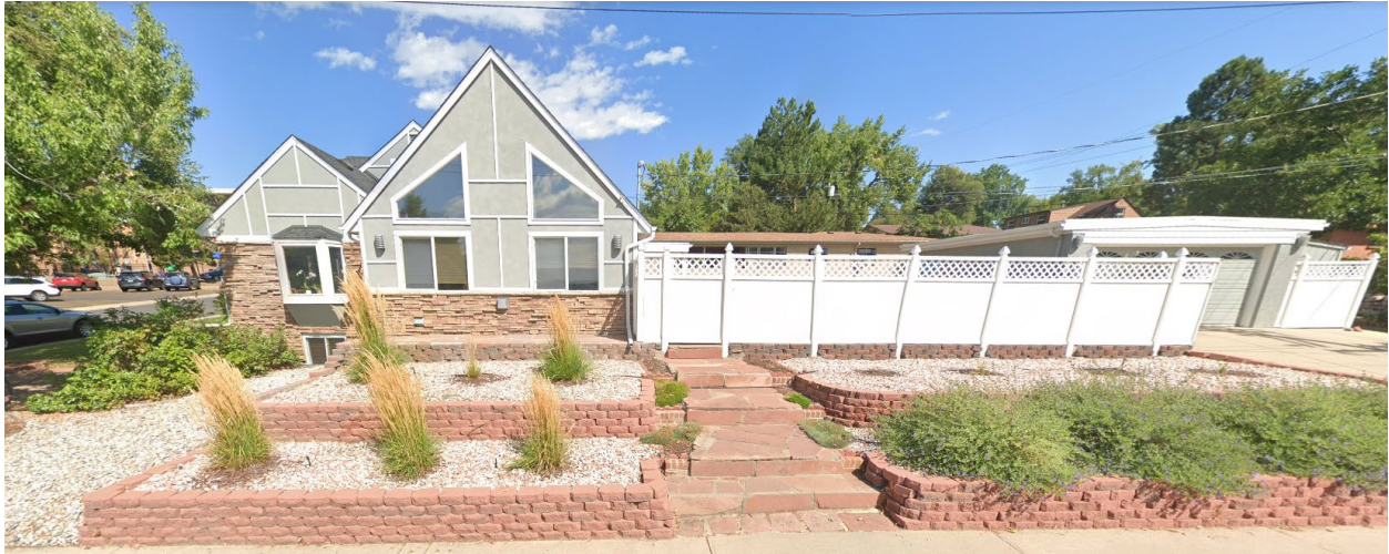
View of the property to the north, across East Dakota Avenue, looking north.
