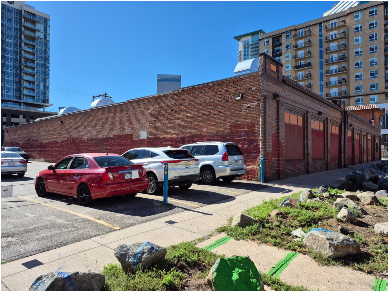
Image 3: California Street Garage, northeast elevation (2025)
