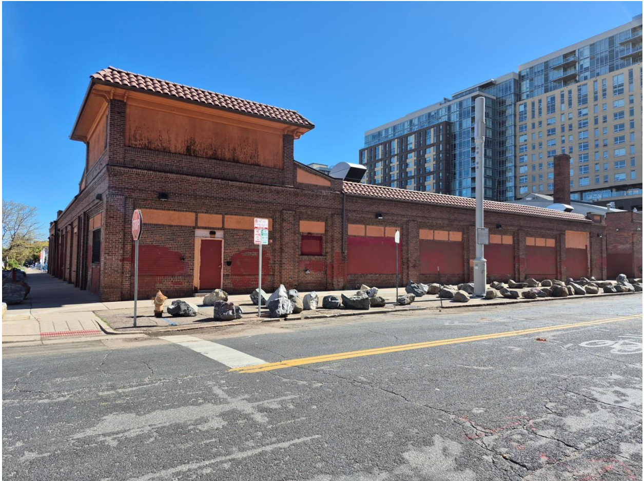
Image 1: California Street Garage, southwest elevation (2025)
