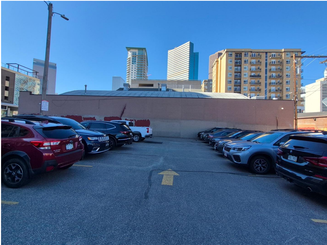
Image 8: Welton Street garage, northeast elevation (2025)
