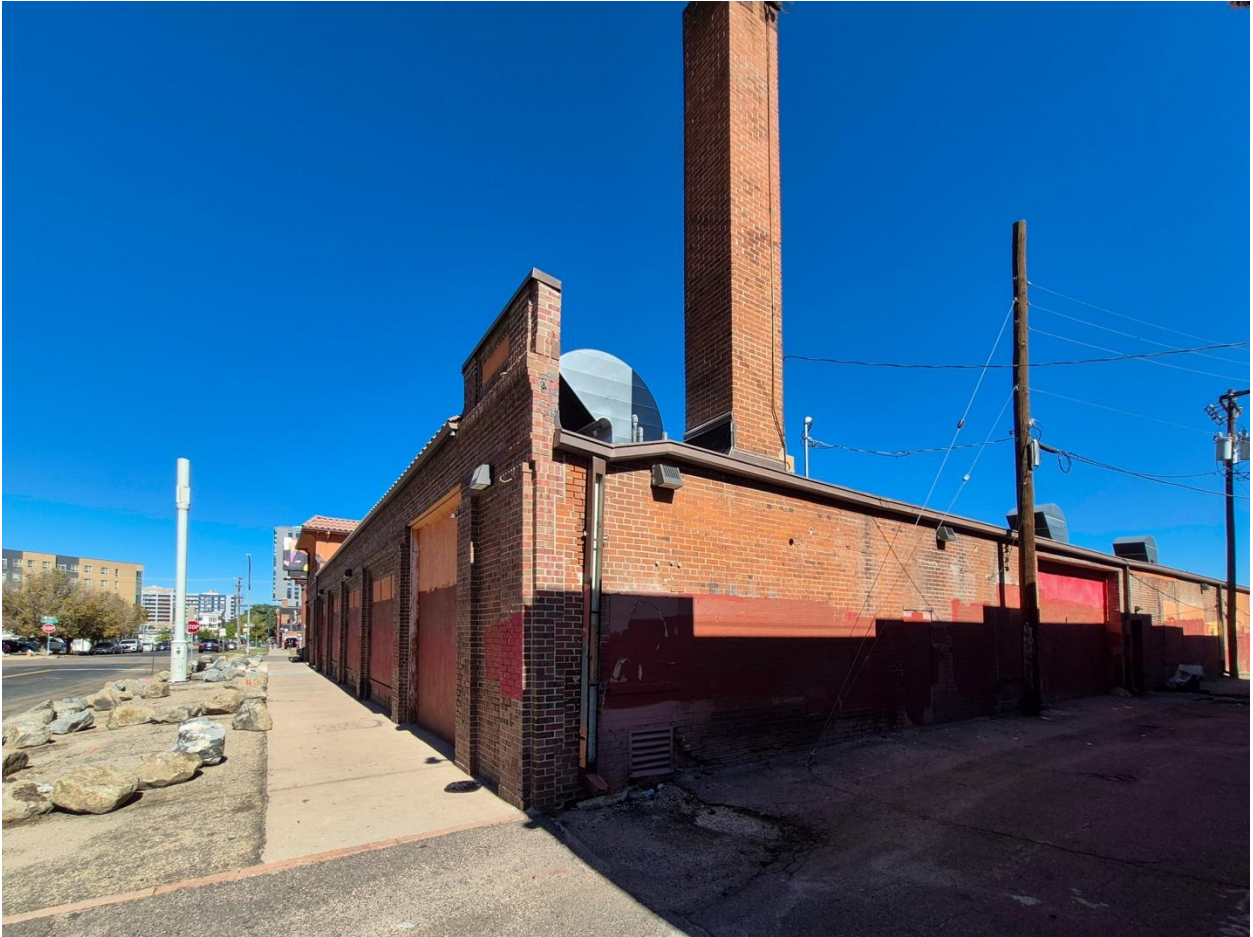
Image 4: California Street Garage, southeast elevation (2025)
