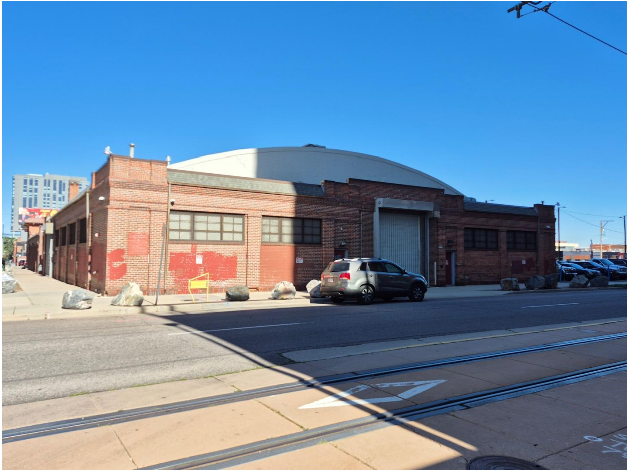
Image 6: Welton Street Garage, southeast elevation (2025)
