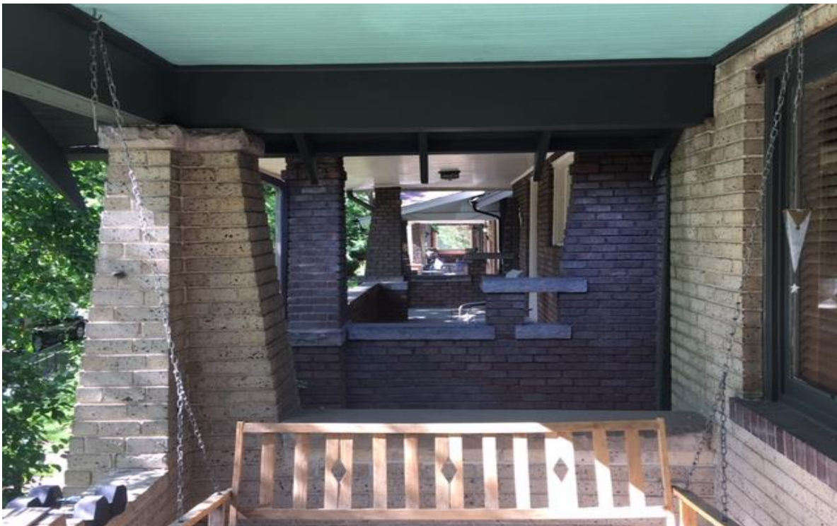
A view through the porches in the 700 block of Steele, demonstrating the Craftsman Bungalow style and form, and the consistency along the block. Photo: David Lynn Wise, 2020.
