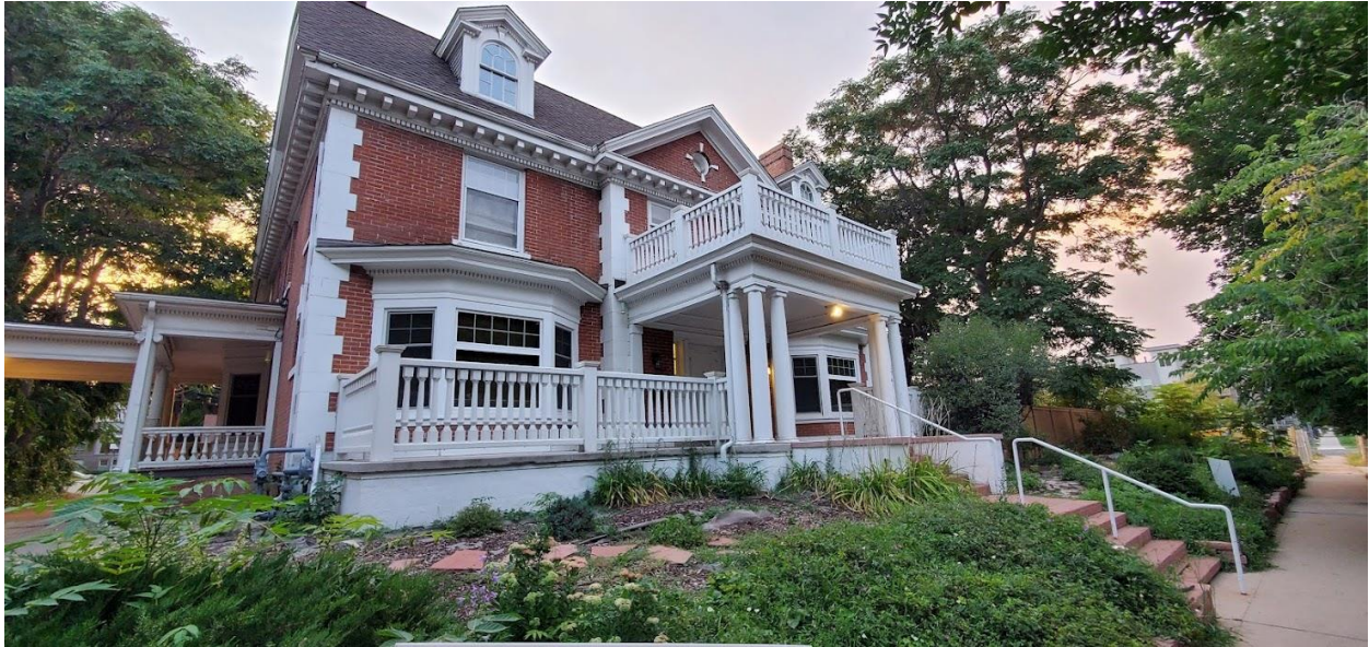
Street level, east side.
