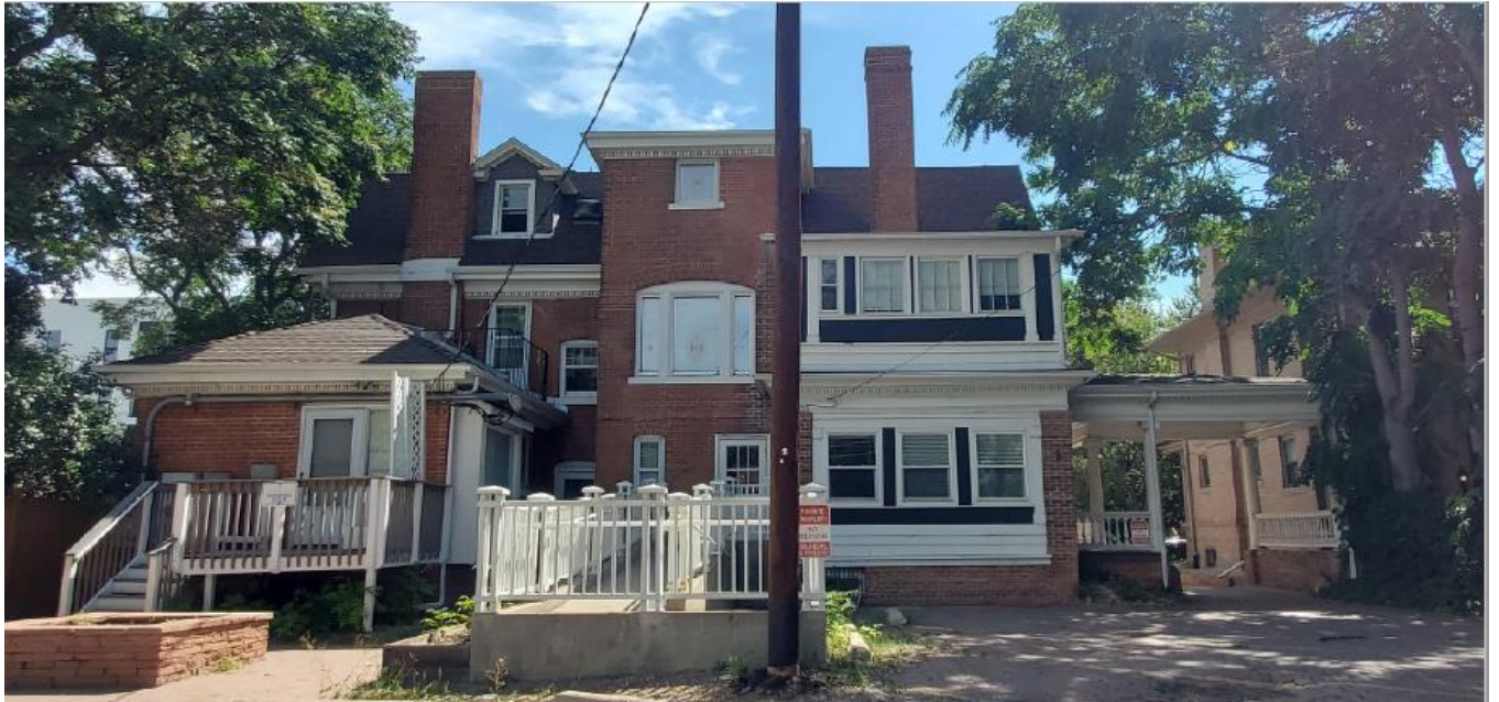
Rear, west side.
