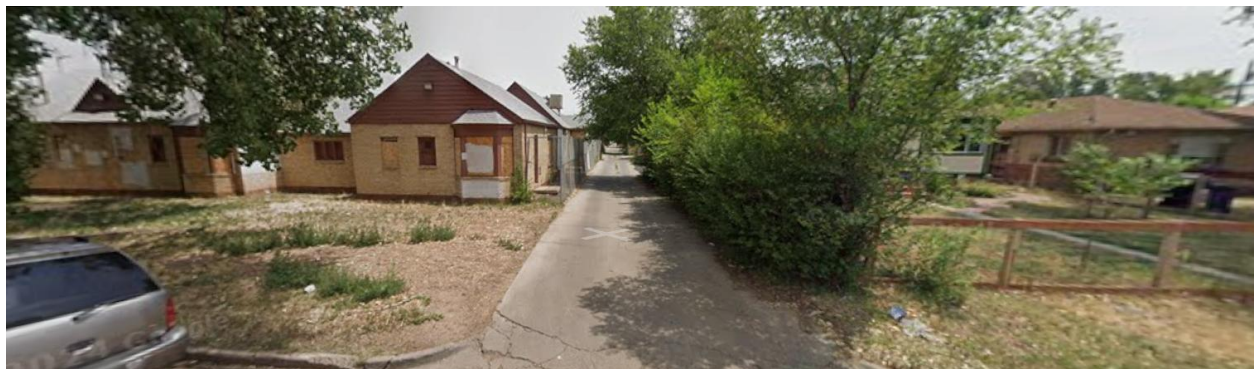
View of the properties to the east across North Wabash Street, facing east.
