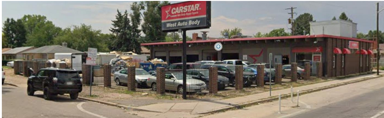
View of the property to the north at the intersection of North Wabash Street and East Colfax Avenue, facing southwest.
