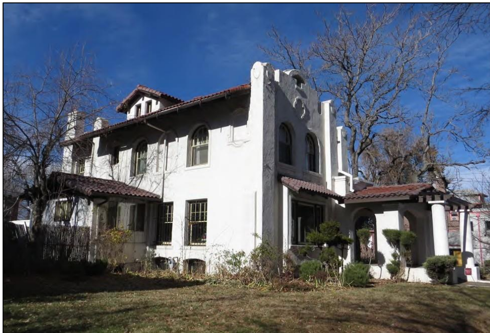
1899 York Street - Ghost/Rose House, South Elevation Photographed by Mason Seymore, 2016
