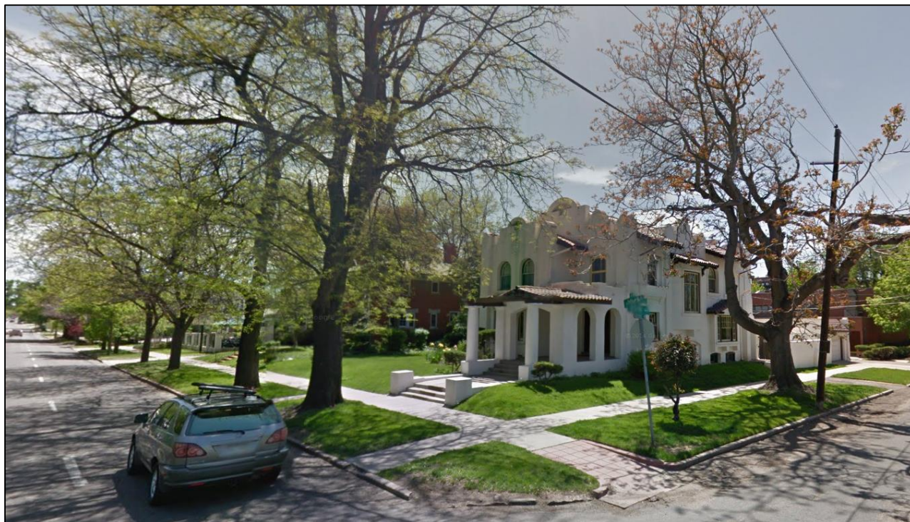
1899 York Street - Ghost/Rose House, West and North Elevations
