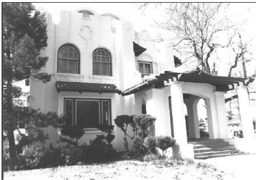
1899 York Street - Ghost/Rose House, West Elevation Photographed by Phyllis Smith, 1973 History Colorado Architectural Inventory Form, 5DV.2721
